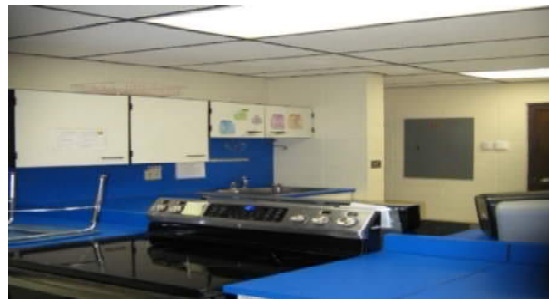
No range Exhaust Hood
