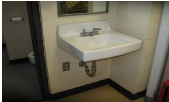
Locker Room Lavatory
