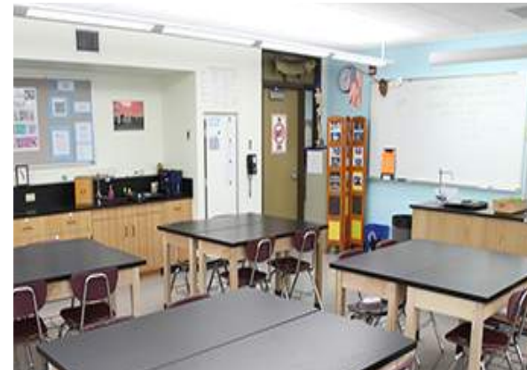
Example of new LED lighting
