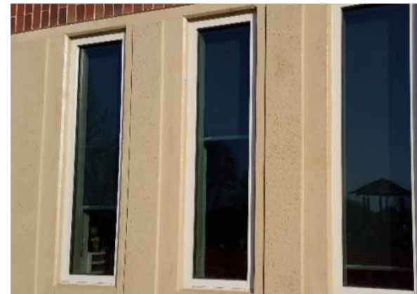
Example of new glazing
