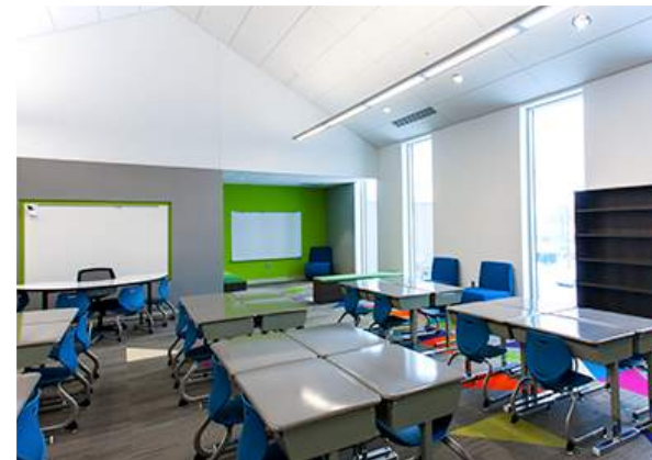
Example of new acoustic ceiling
