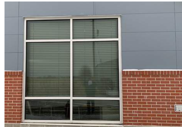
Example of new thermally broken window
