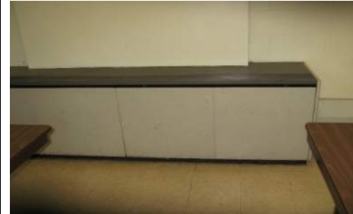
Through-the-wall Unit Ventilator
