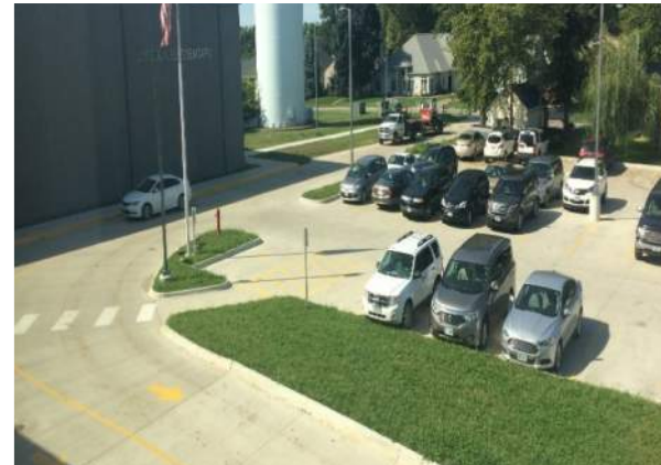
Example of new paving
