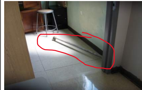
Pipe in Middle of Floor
